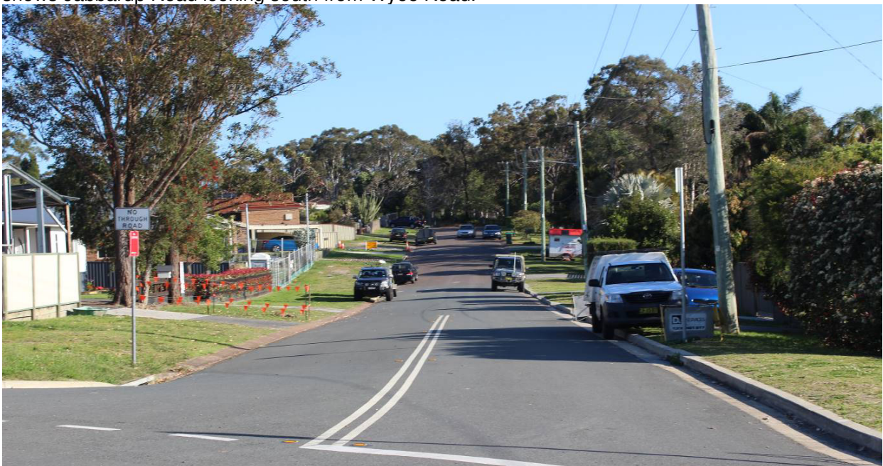
Photograph 5 – Jabbarup Road looking south from the intersection with Wyee Road.
