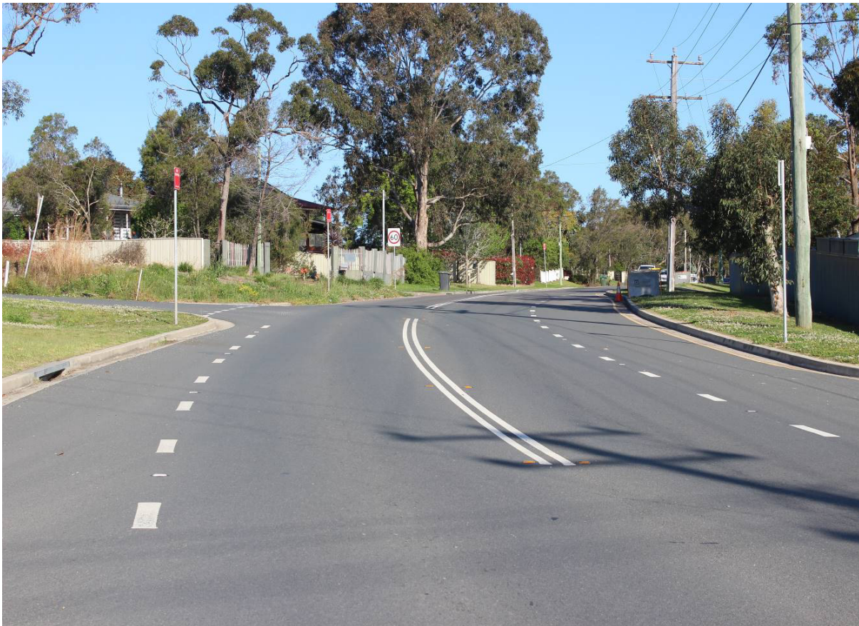
Photograph 3 – Wyee Road east of Gosford Road intersection.
